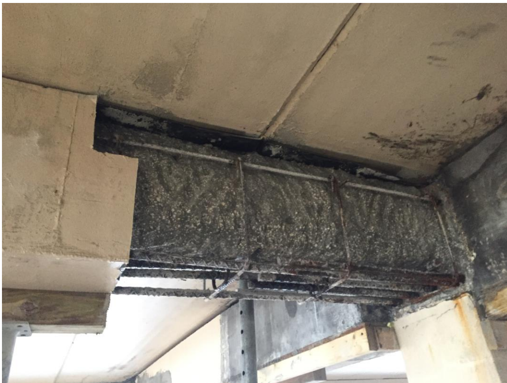
Picture 2: Typical garage excavation inspected
