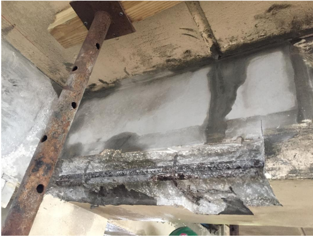
Picture 1: Typical garage excavation inspected
